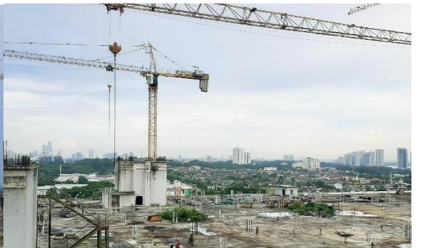
Tower D : Serviced Apartment
