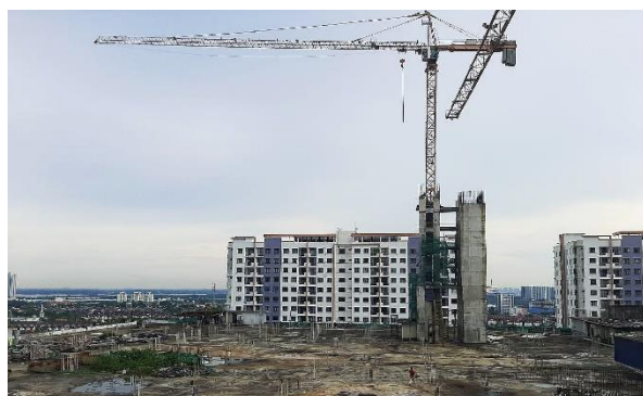
Tower E : Serviced Apartment
