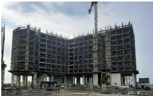
Tower B : Serviced Suites
